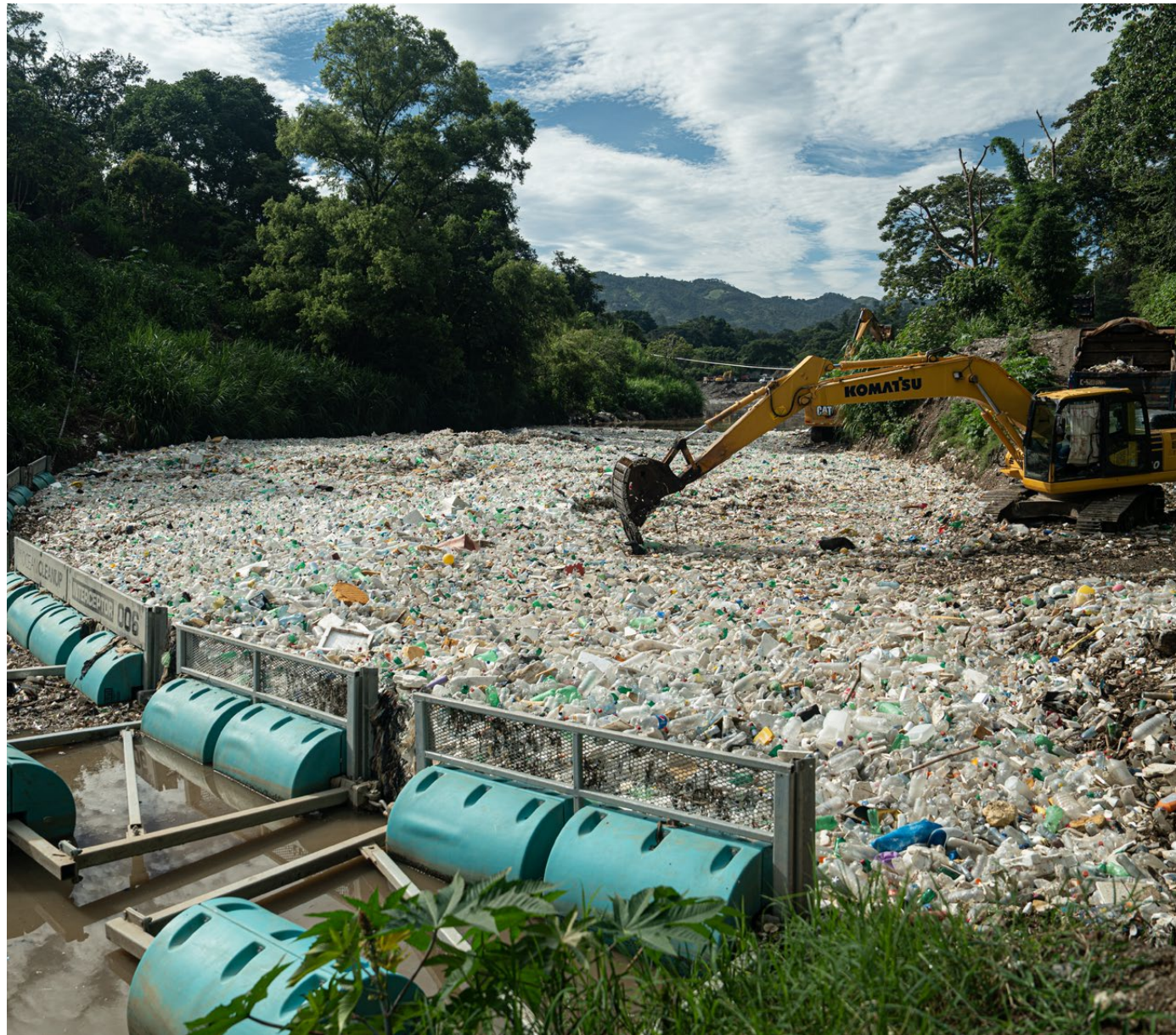
Credit: The Ocean Cleanup – Excavators removing trash from the Interceptor Barricade in Guatemala, Rio Las Vacas (July 2023).
